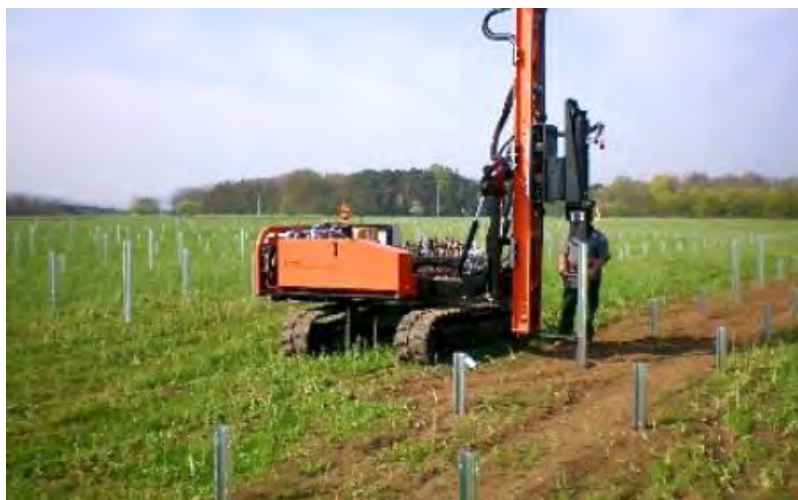
Figure 9 – Typical Low Ground Pressure Screw Pile Vehicle
